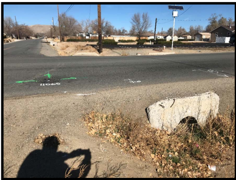
Figure 8 – Culvert crossing E. 4 th Avenue
